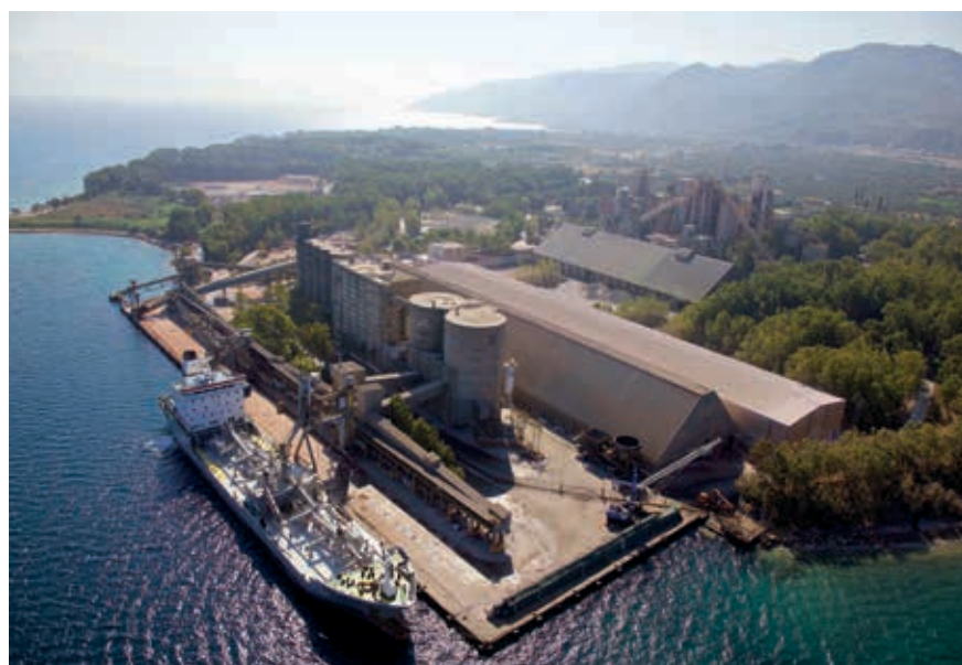
Patras cement plant, Greece
