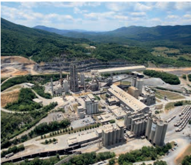
Roanoke cement plant, USA
