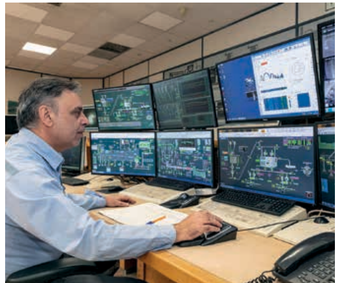
Kamari cement plant, Greece
