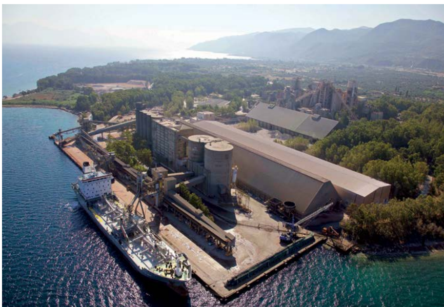
Patras cement plant, Greece
