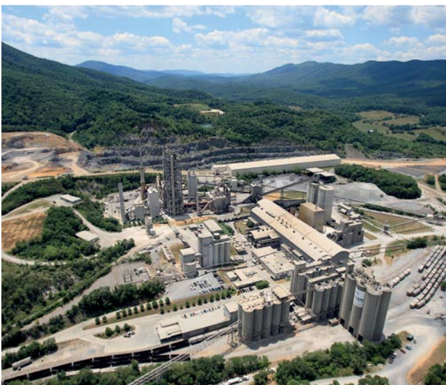
Roanoke cement plant, USA
