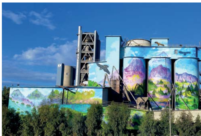
Thessaloniki cement plant, Greece
