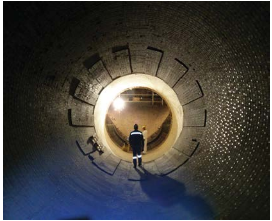
Kamari cement plant, Greece
